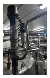
The radial seal design of the D4 Series reduces the loss of valuable yoghurt mix to drain during valve opening/closing which saves costs and provides a cleaner operating environment. Reduced CIP losses to drain, low actuator air consumption (5 bar/72 psi), and no compressed air supply required for valve removal and maintenance will help to further generate utility cost savings for the customer in the years ahead.
